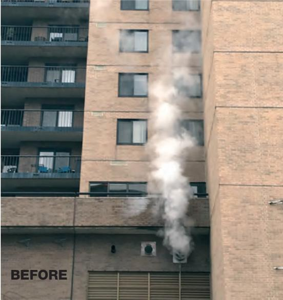
The exhaust plume is creating ice build-up and potential deterioration on the wall. And is a nuisance to the residents.
